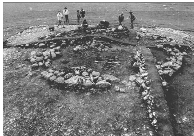
Fig 2.18 Excavations at Hardendale Nab, Cumbria (OA North).
